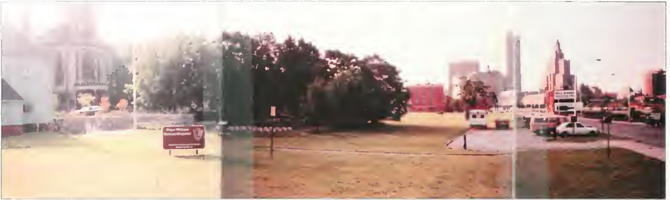
Figure 1.52. Panorama looking south from Smith Street taken in July 1981 following completion of Phase I that included construction of the ramp-stair structure, visible at the south (right) side of the Antram-Gray house. This photograph also shows the initial improvements made between 1976 and 1979, including renovation of the house with its rear shed addition, the gravel parking lot, sign, and seeding of the site. The grove of trees are the Norway maples planted in Bernon Park in 1953. (Roger Williams National Memorial archives.)
